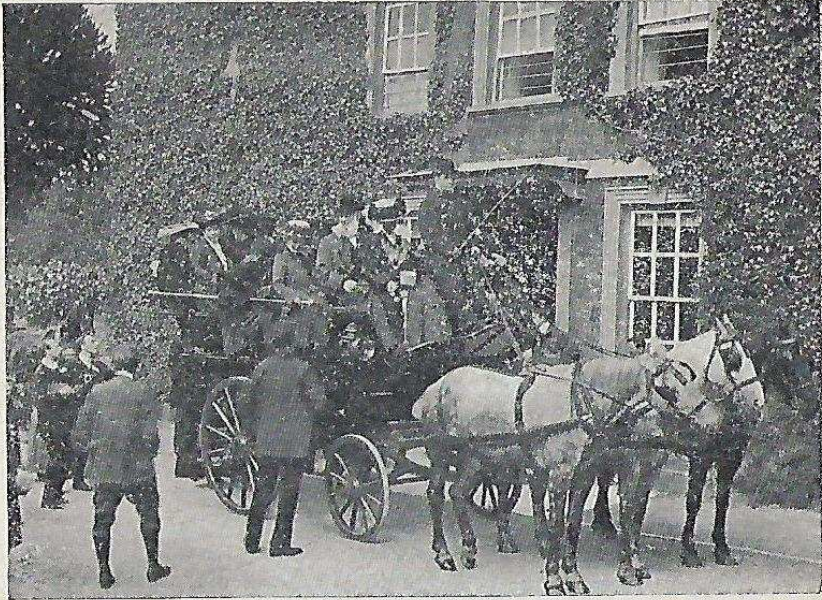
Transport as it was before the first world war: a wagonette leaves the Friends' School at Sibford (the part of the building shown is the original Charles I mansion).
